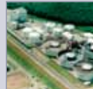
WASTE WATER TREATMENT PLANT
